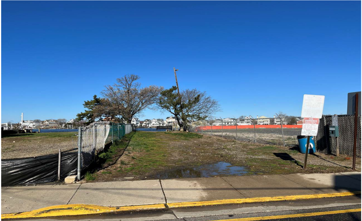
Existing Borough Boat Launch
