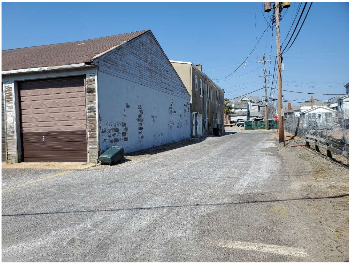
Photograph facing north from the north portion of the site, showing Poppi Place and an adjacent industrial building proposed to be demolished.
